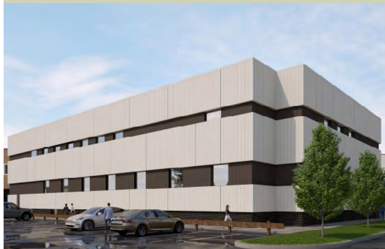
Bethesda Regional Health Centre à Steinbach
